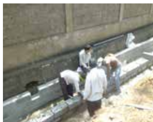
Drain construction in Siltara
