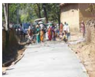
RCC road construction in village
